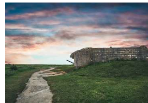
Following the invasion of the USSR and the United States' entry into the war alongside the British, German strategy in the West shifted from offensive to defensive. Hitler ordered the construction of a line of fortifications along the western coast capable of repelling any Allied invasion attempt. Construction of the Atlantic Wall began in early 1942.
